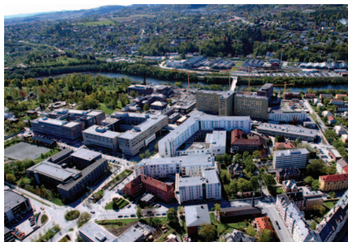
St. Olavs Hospital. Under construction
