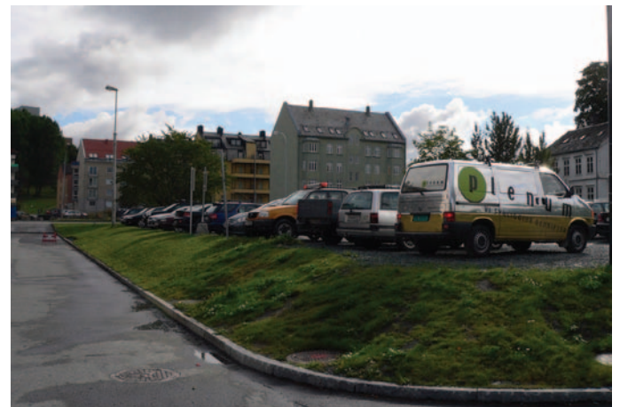
Looking south-east towards the building site over Elgestergate.
