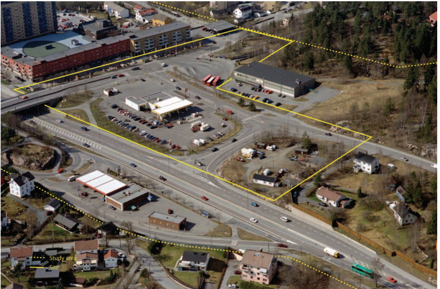
Looking north-west towards the site.
