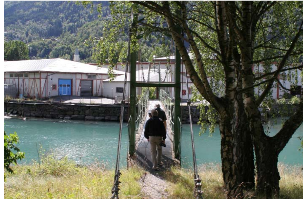
Suspension bridge across the river
