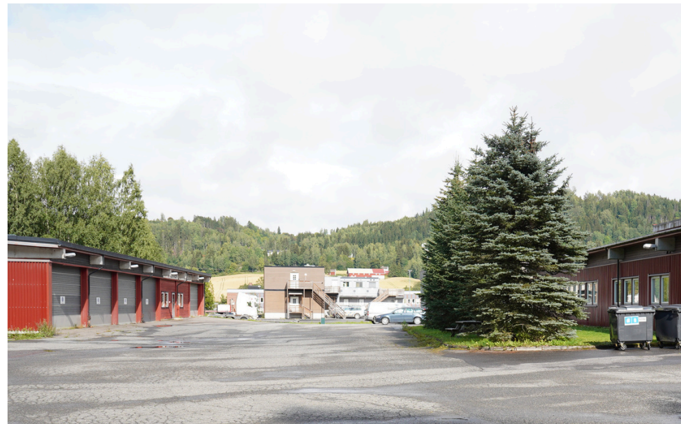
Fire department and doctors offices. The temporary offices of the national road agency (Statens veivesen) can be seen in the back.
