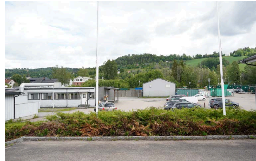
Recycling station at the Lupro site.
