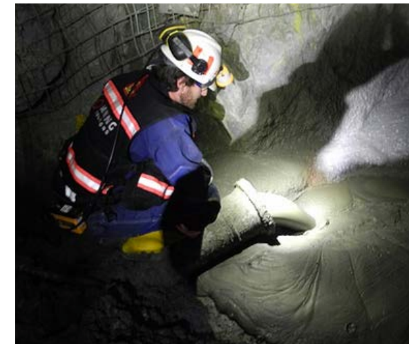
Underground Backfill. Photo: Sika Canada
