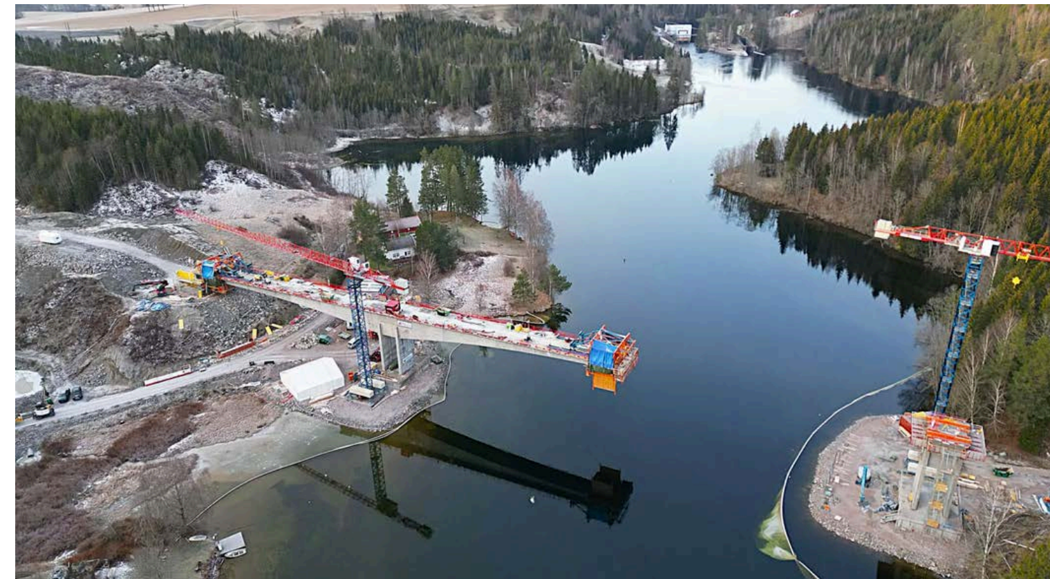
The new bridge along fylkesvei 359 is under construction and is set to open later in 2025. Photo: Olav Heggernes/Telemark Fk
