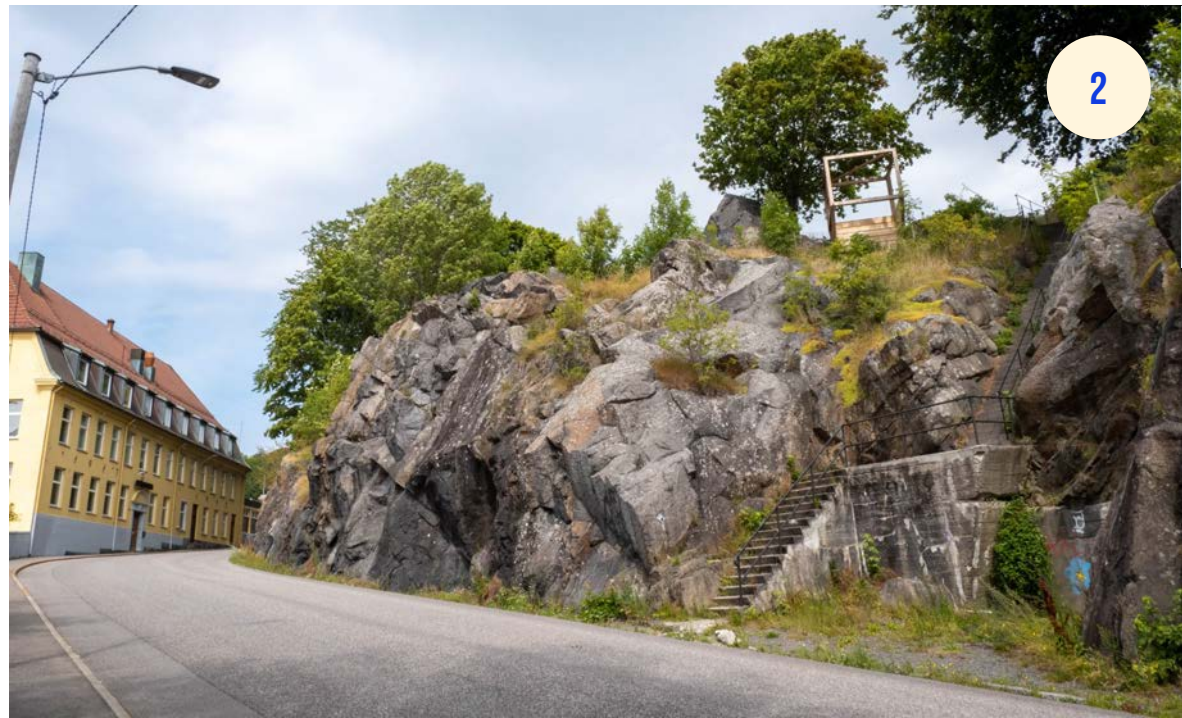
The Road along Bøkkerfjellet and staircase leading up from the west. The Farris factory is to the left.
