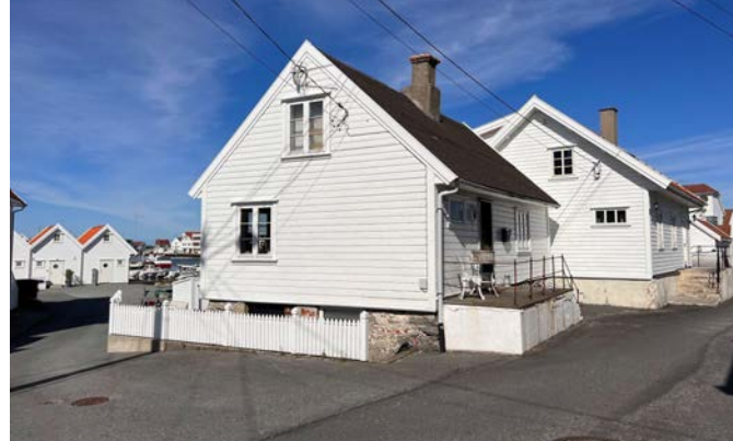
Narrow and disconnected sidewalks
