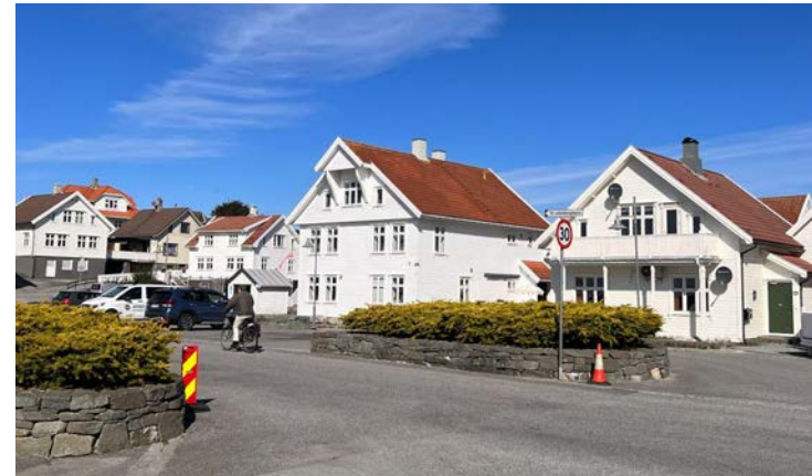
5. Strandveien is characterised by a valuable grouping of wooden houses
