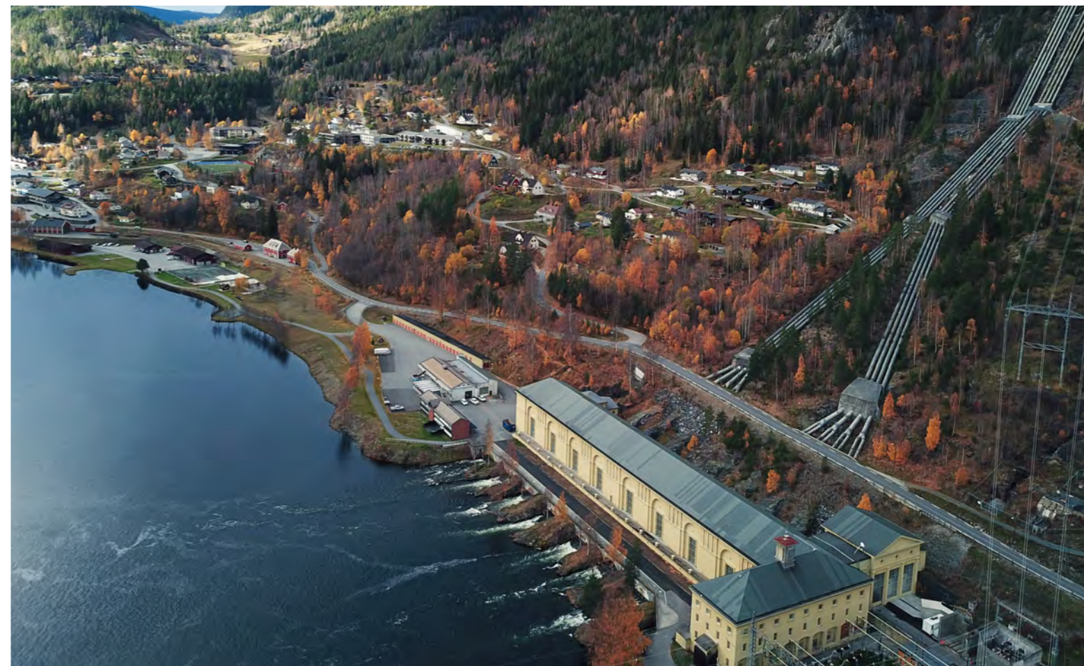
The hydro power plant Nore 1 and the pengates make a powerful imprint on Rødberg.
