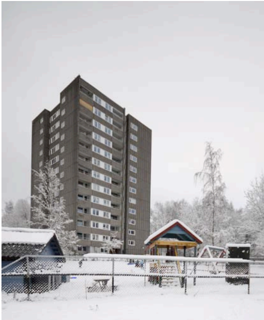
Tower residences east of the project site.
